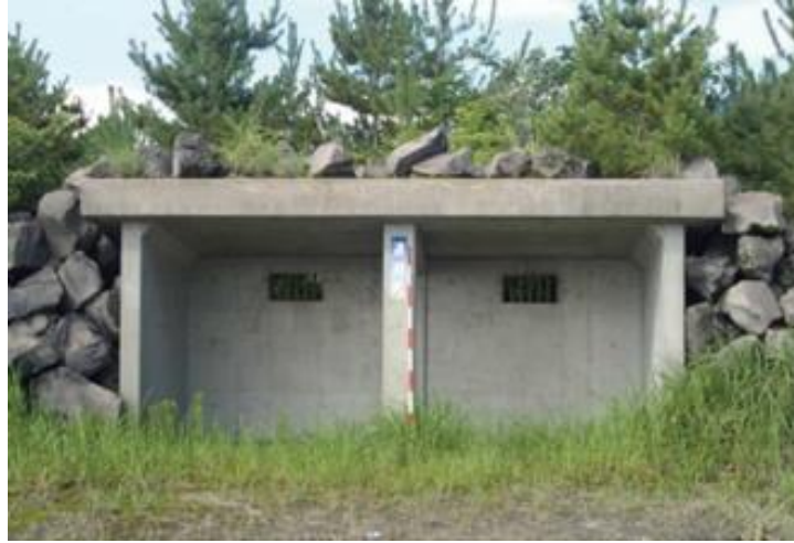
[退避壕設置事例（桜島）]
